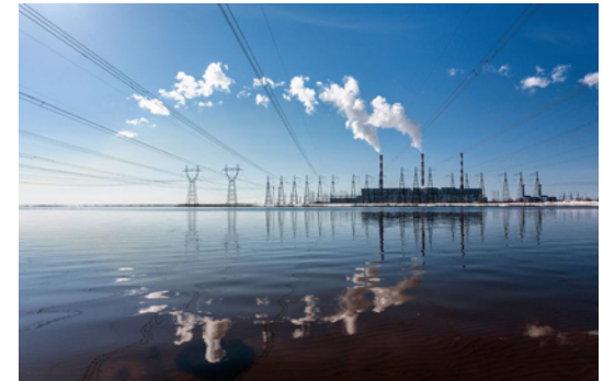
Surgut state district power station (GRES-2)
