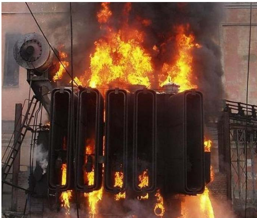
Fig. 1 – Transformer failure resulted in a fire
