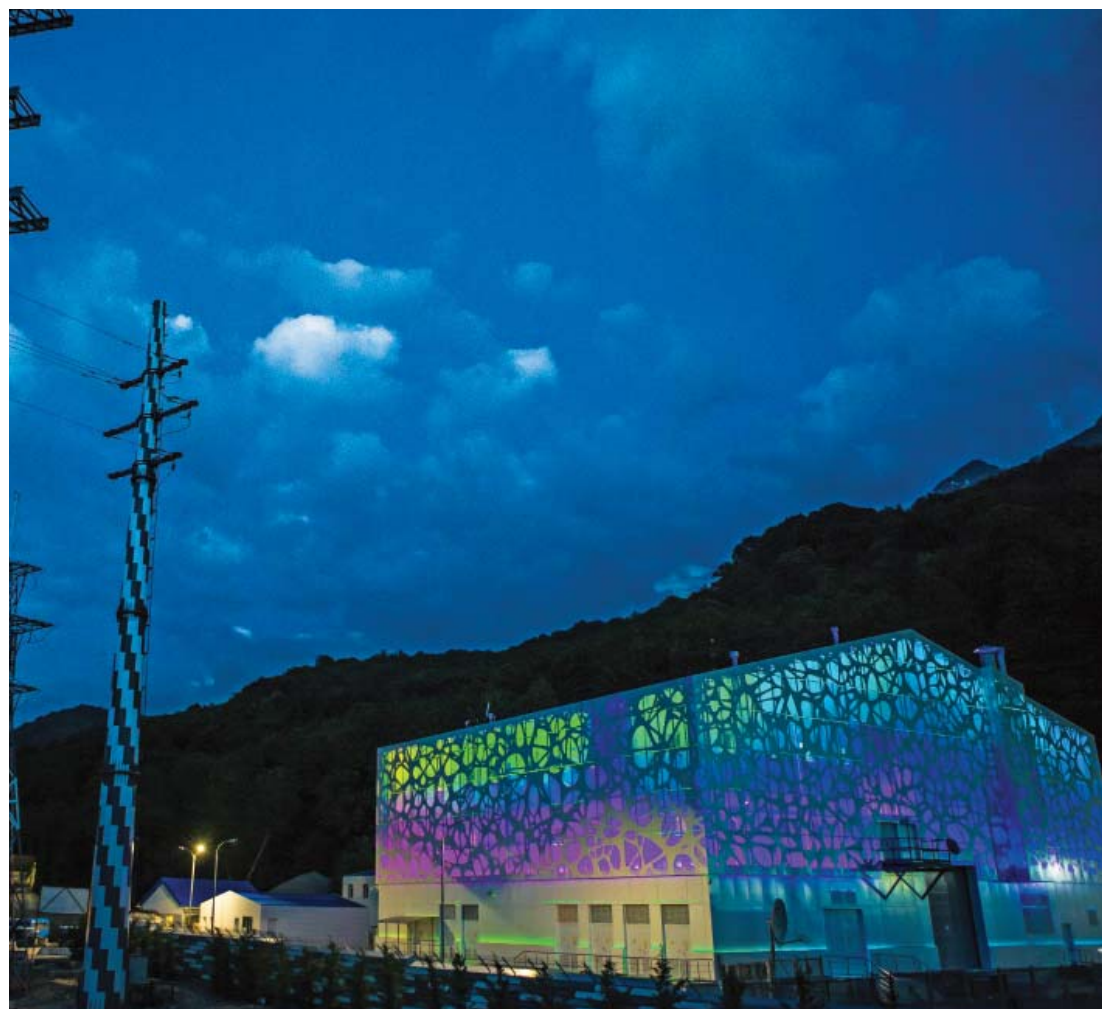
Poselkovaya 220kV substation in Krasnodar Territory is one of seven FGC UES facilities where telecontrol is already implemented
