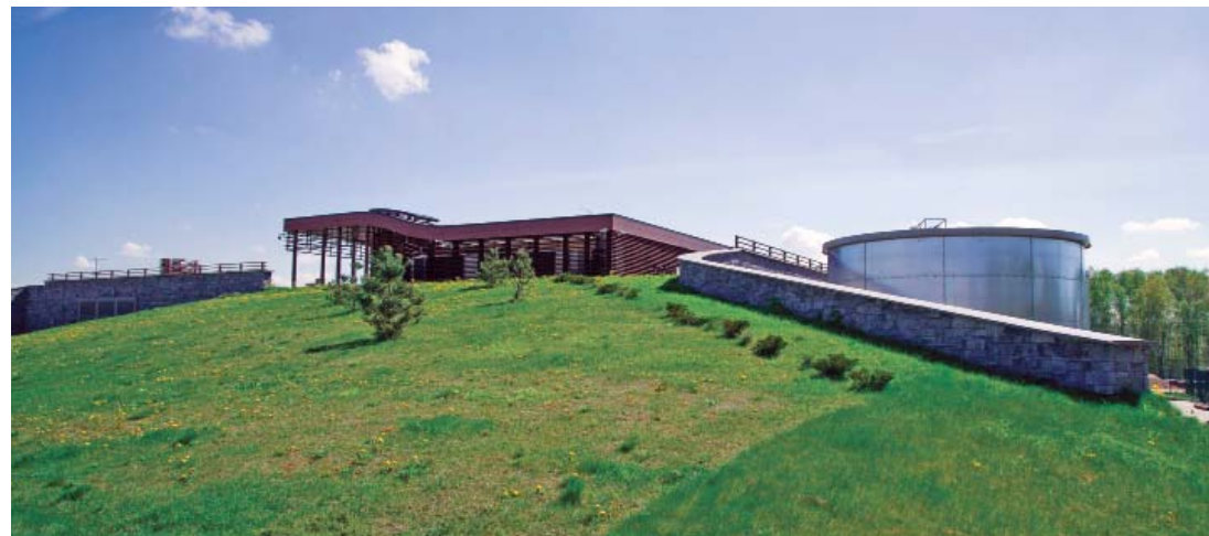
Fig. 2 Skolkovo 220kV underground substation involved in electrical power supply
