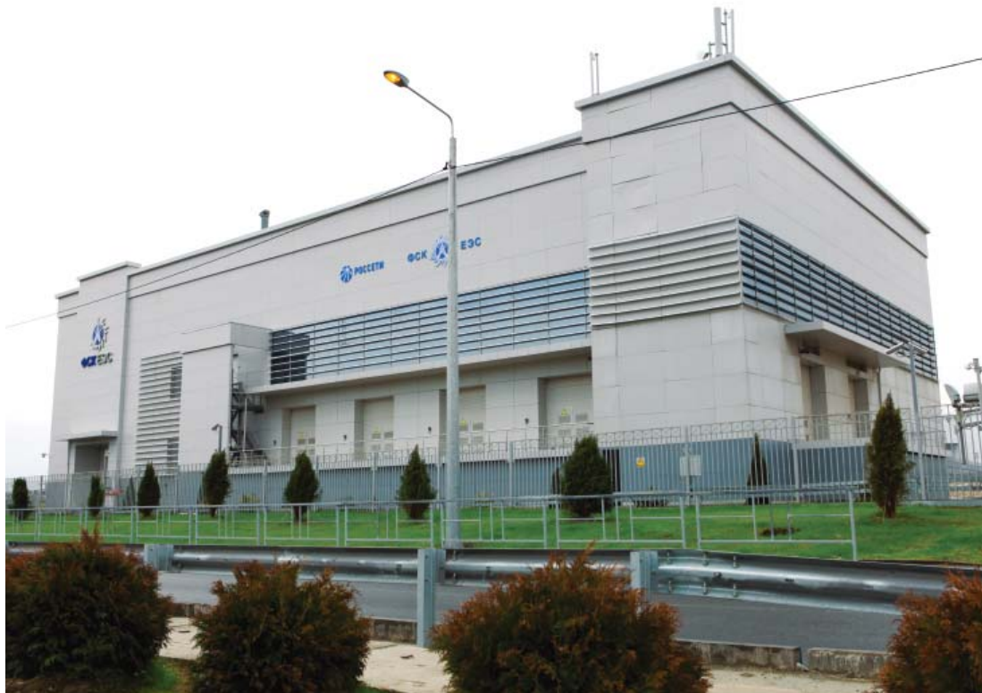
Substation 110 kV Imeretinskaya
